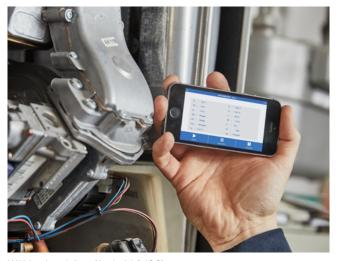
Wöhler A 450 App (Android & iOS) Displaying the measured data on a mobile device.
