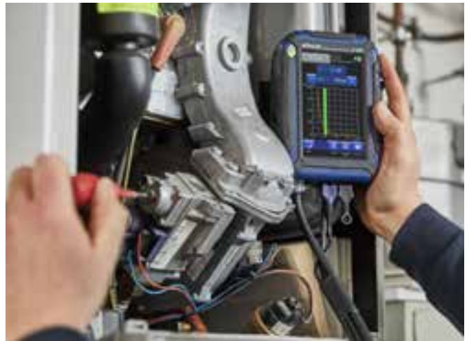
The tuning guide offers an advanced guidance to properly adjust the burner.
